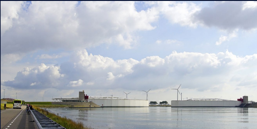
The Maeslantkering closing the Rotterdam waterway against a surge · Photo: kees torn, CC BY-SA 2.0
